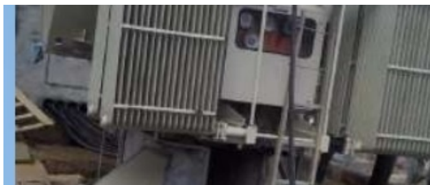
Transformer oil filtration - 2.5 MVA, 33 kV - Bharat Electronics Limited, Muradnagar
