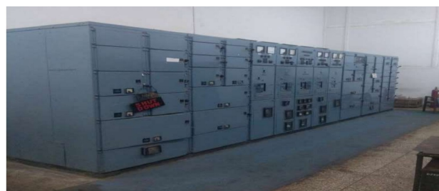
LT panel repair & services - Ram Nagar, Uttarakhand
